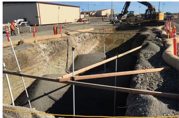
*Travis Air Force Base built the first ever subgrade biogeochemical sulfate reactor that relies on sulfate reduction to biologically treat petroleum contamination in soil and groundwater.*
